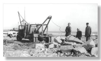
Bill used his utility truck for many things: hauling boats, picking up moorings, and general odd jobs. It had an "A" frame boom over which a cable ran to the truck's winch. 1952 photo from the RYC archives
